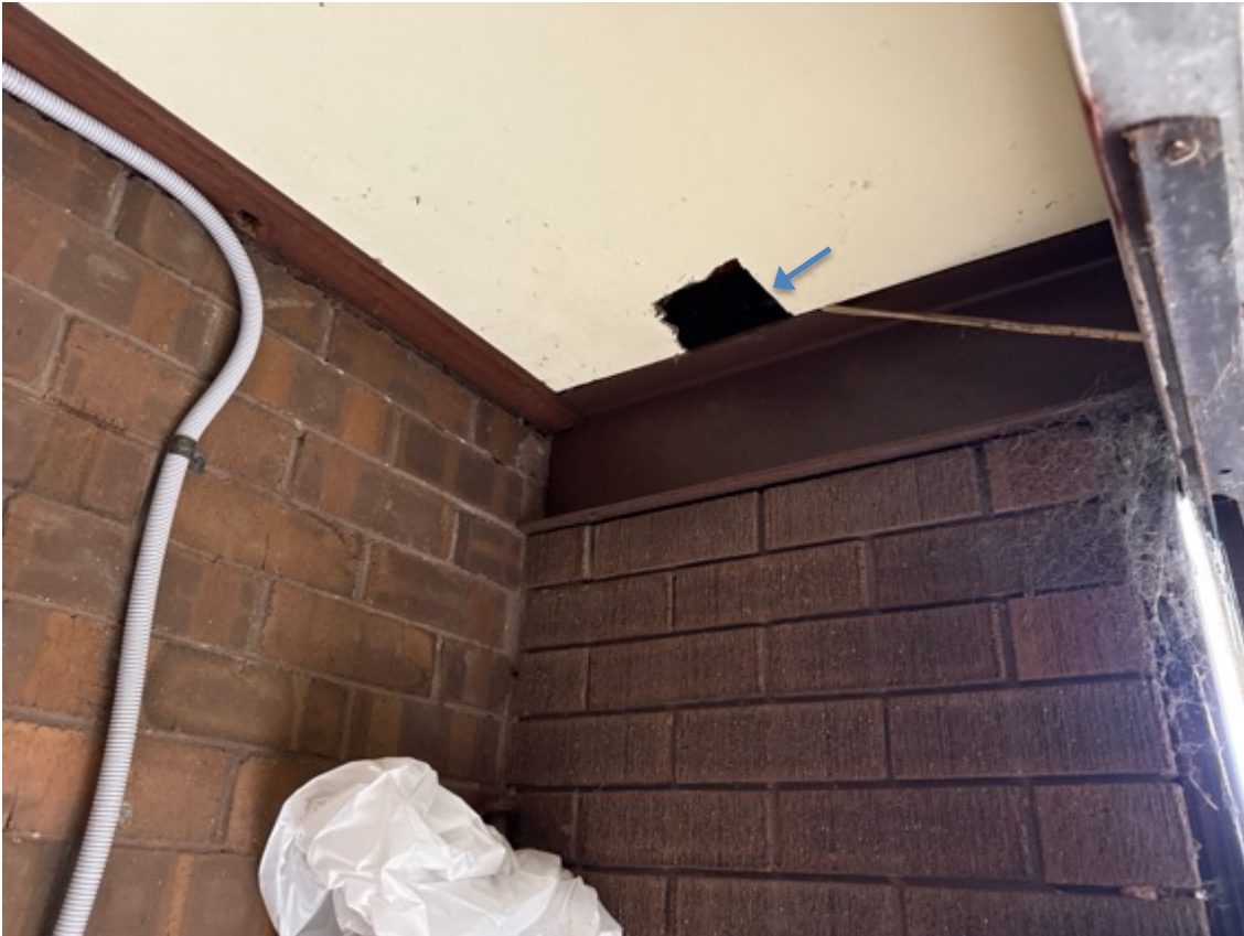
Plasterboard displays imperfections and sections require patching (consistent with age.)
