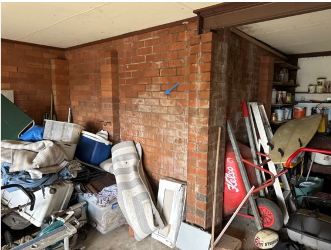
Garage brickwork displays efflorescence.
