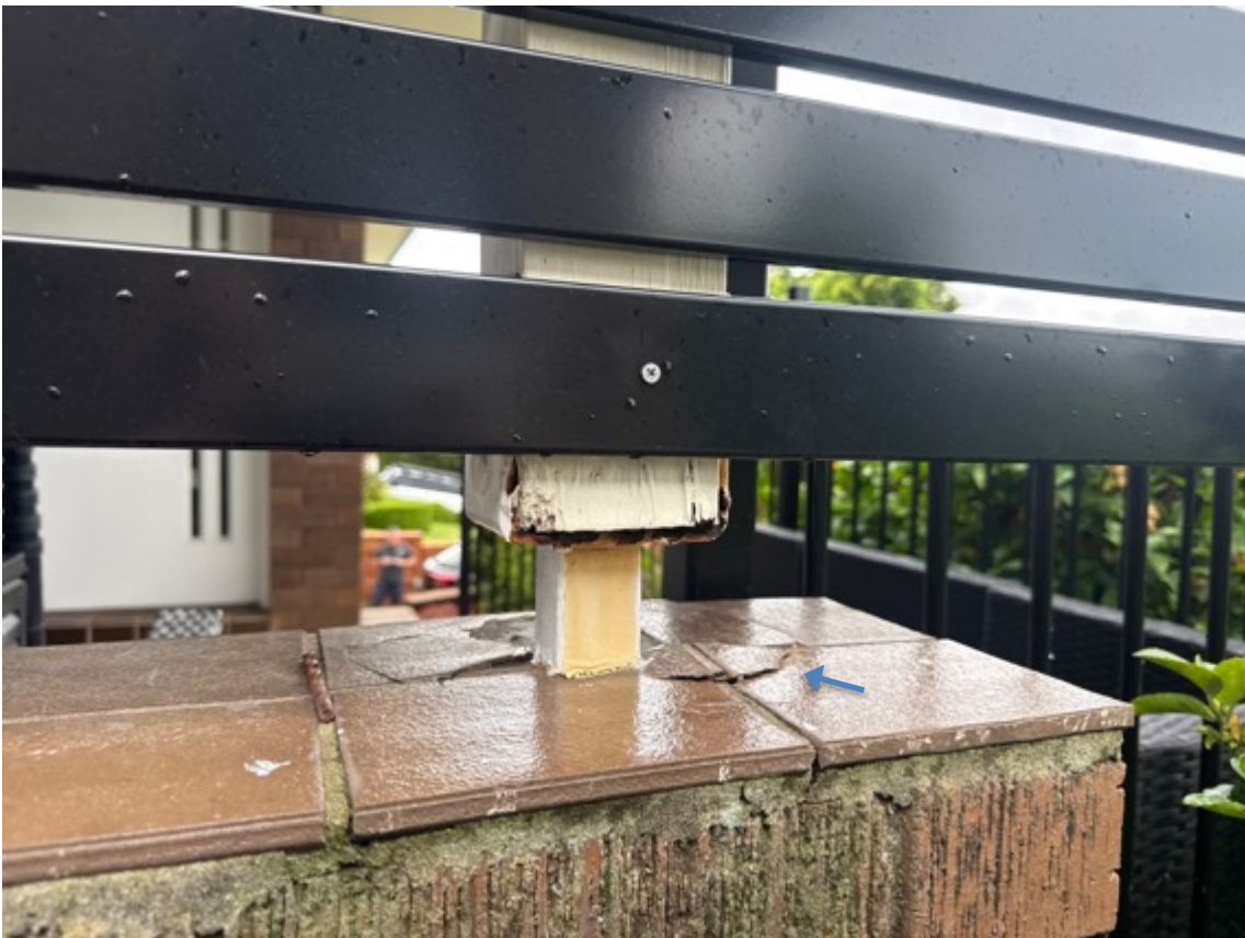
Isolated sections of external tiles are cracked, consistent with age (front left elevation example above.)
