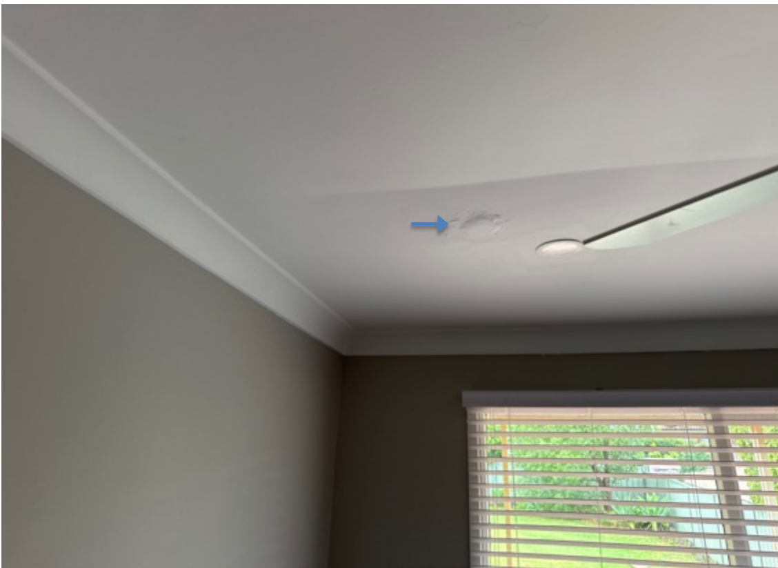
Rear right side bedroom plasterboard displays imperfections and has been patched here.
