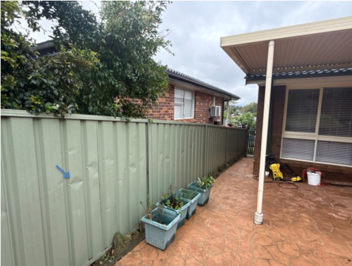
Site fences are in serviceable condition, isolated sections are dented and leaning - consistent with age.
