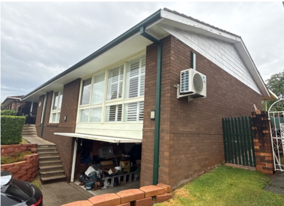
Exterior timber displays moderate level weathering and surfaces are paint blemished - consistent with age.
