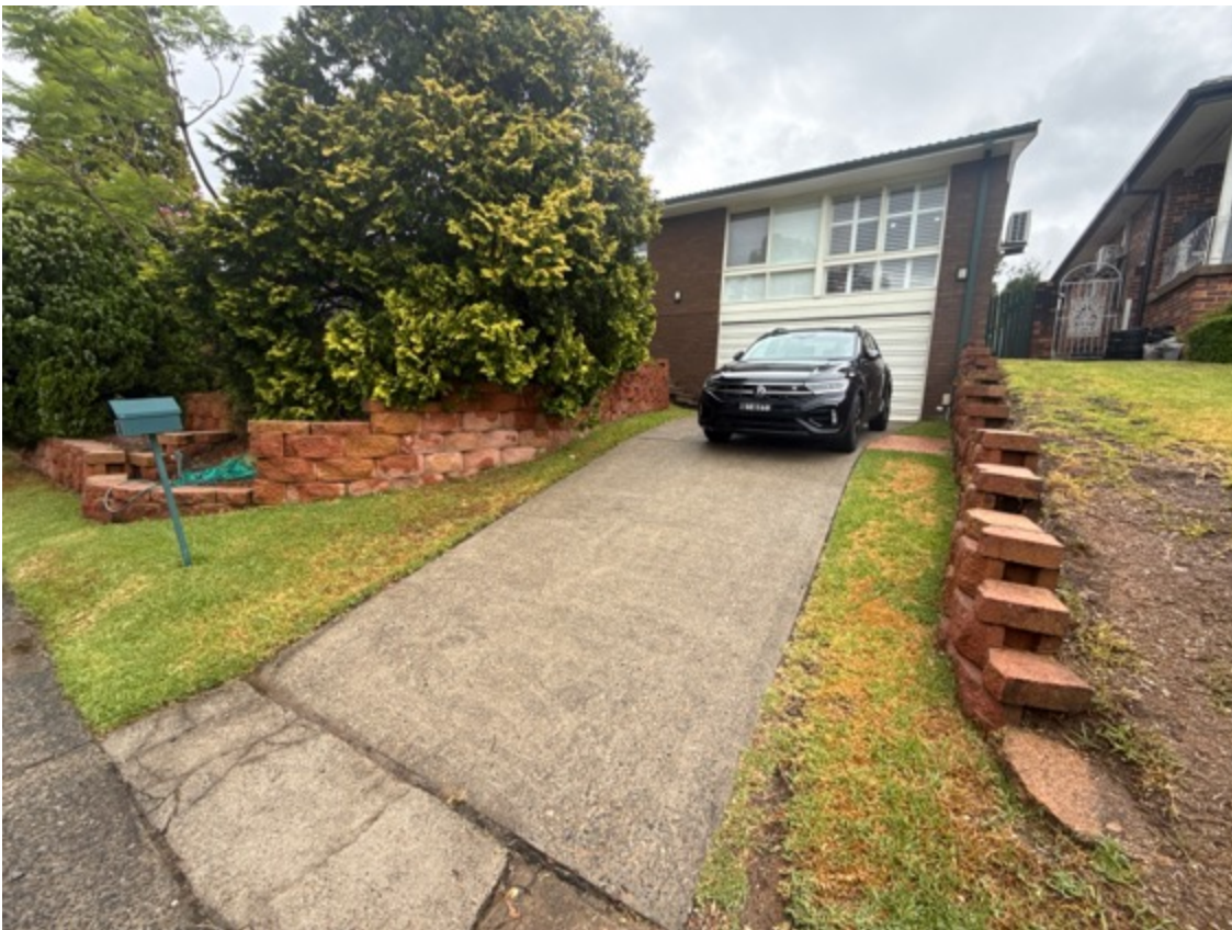
Exterior concrete presents in satisfactory condition for the age, isolated sections displays shrinkage cracks and undulations - consistent with age.
