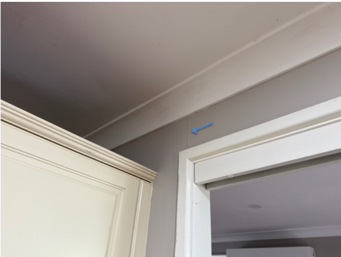
Isolated sections of plasterboard and cornices are cracking (example kitchen area above.)
