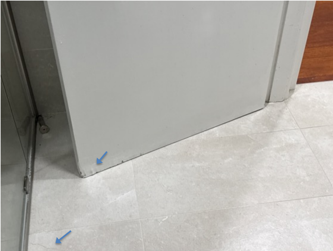
Isolated sections of tiles are cracked and the door is frayed at the base, consistent with age.
